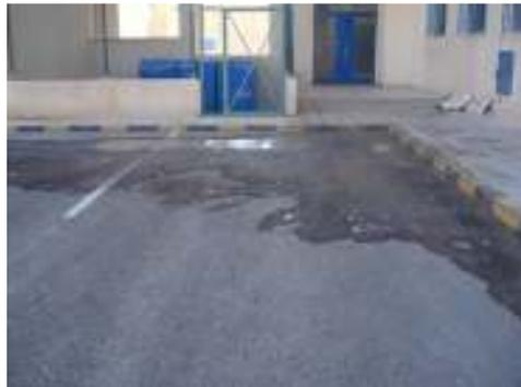
**Figure 4. No Proper Drainage in this corner.**
